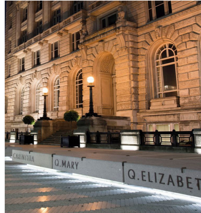
Under seat lighting with LED strips, the downward direction of the reduces light pollution.
