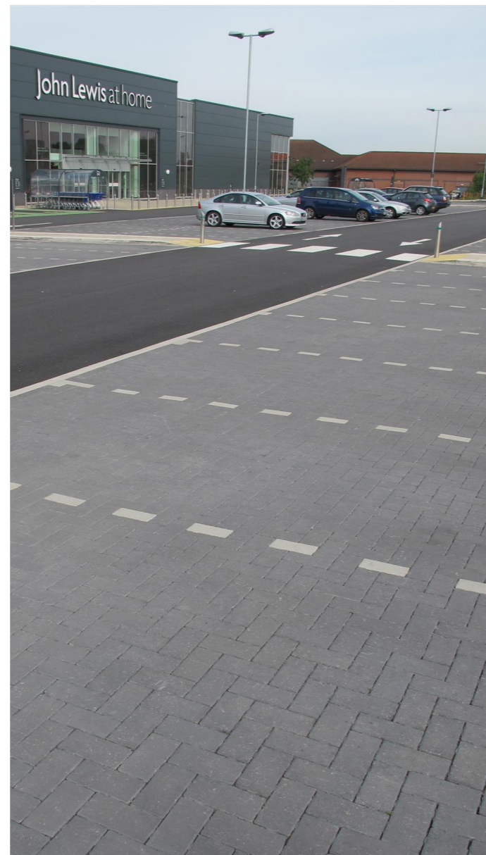
The John Lewis store in Tamworth has hydro-paving, laid out so that the parking lines and the parking spaces are defined.
