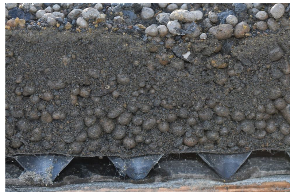
Green roof substrate cross section
