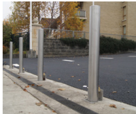
Bollards | Site Wide Removal Bollard
