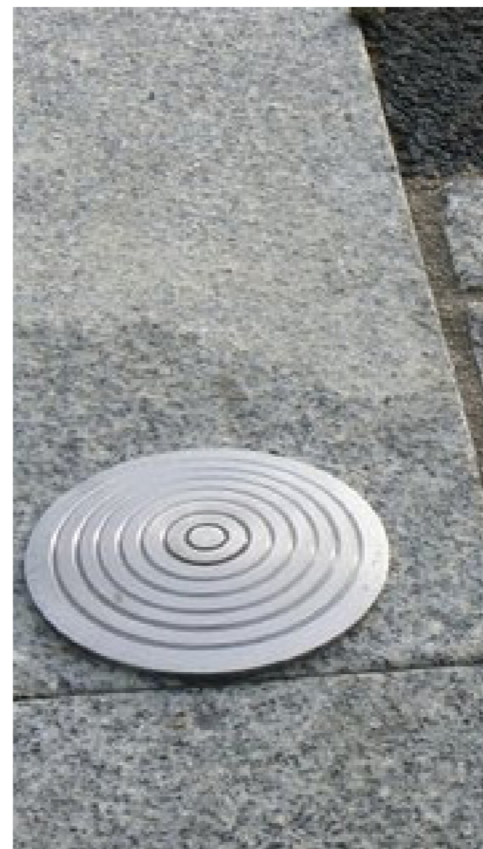
Demarcation studs are used in Durhamgate to show the edges of the car park.
